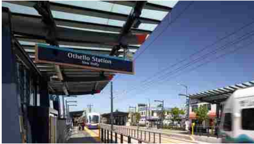
Image 7: LINK Light Rail Othello Station on MLK Jr. Way at NewHolly
